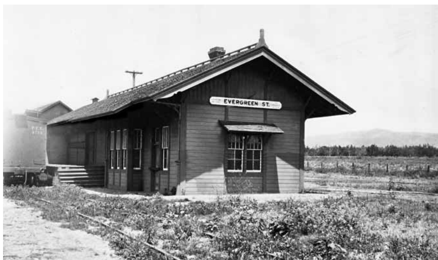
This Common Standard No. 7 passenger and freight depot was built at Evergreen St., MP 502.2, in 1888. It was later converted into Packing-house for the Southern California Fruit Exchange. —SP photo, courtesy Western Railway Museum
